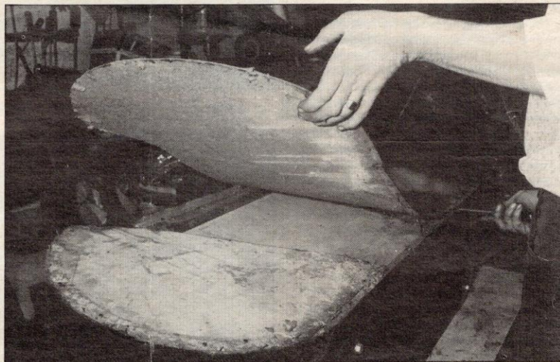
Old panelling is removed carefully as it will be needed for patterns
